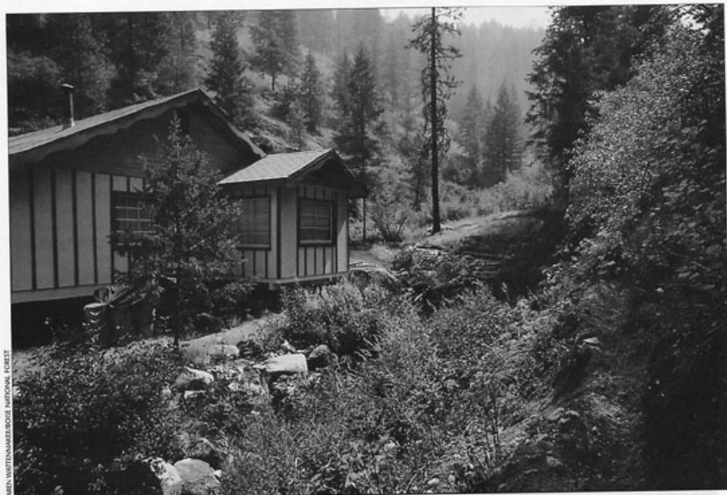
Nestled on private land in the Star Gulch Fire area of the Boise National Forest, this home (above) is protected by defensible space, a foam-treated roof, and a fireline—a deep trench that fire is unlikely to cross. Left, this thickly forested area of Strawberry Creek in Boise National Forest was the site of an undefended house that could not be saved.
